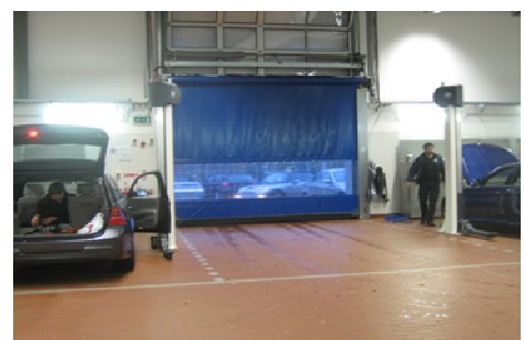
Fast acting doors, like these, keep the heat in. They are activated by below-floor sensors
