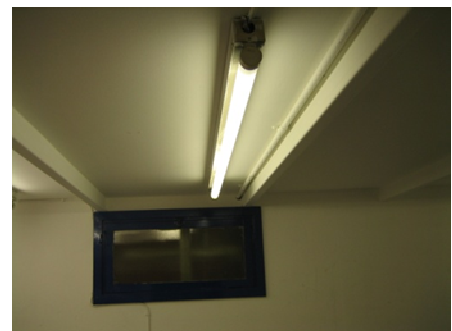
Replace T12 fluorescents for T5 ones
